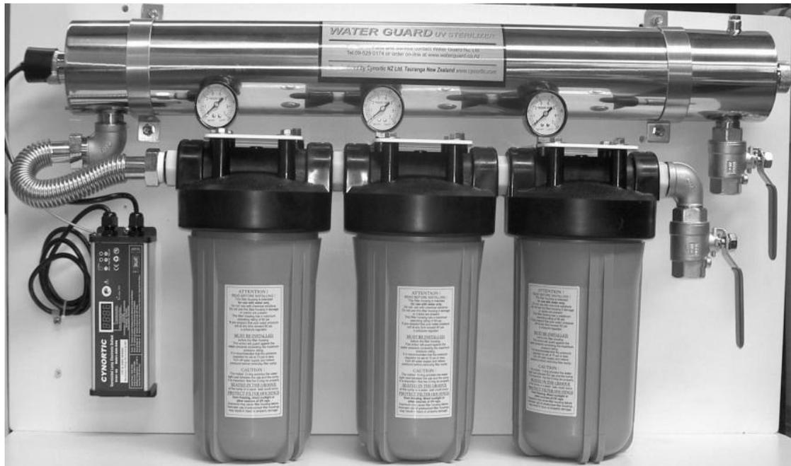
[7] The water comes in the pipe at the bottom right, goes through the plastic filters shown and then through a metal hose to the top steel cylinder which contains an element emitting ultra violet light, before emerging for use at the pipe at the top right. The electricity is supplied by a device known as the ballast, shown to the left
